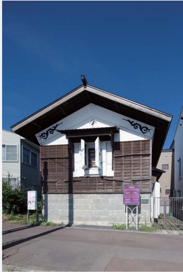
Location: 15-3 Sumiyoshi-cho, Otaru Built: Early Meiji Period Structure: 2 story clay building
